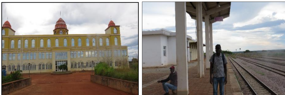
Figure 4-51: CFM station at Jamba
